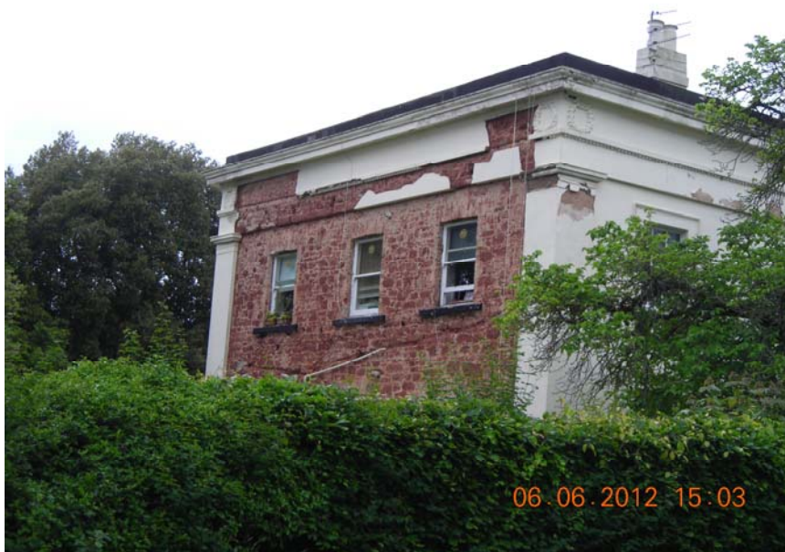
South east elevation showing removal of render
